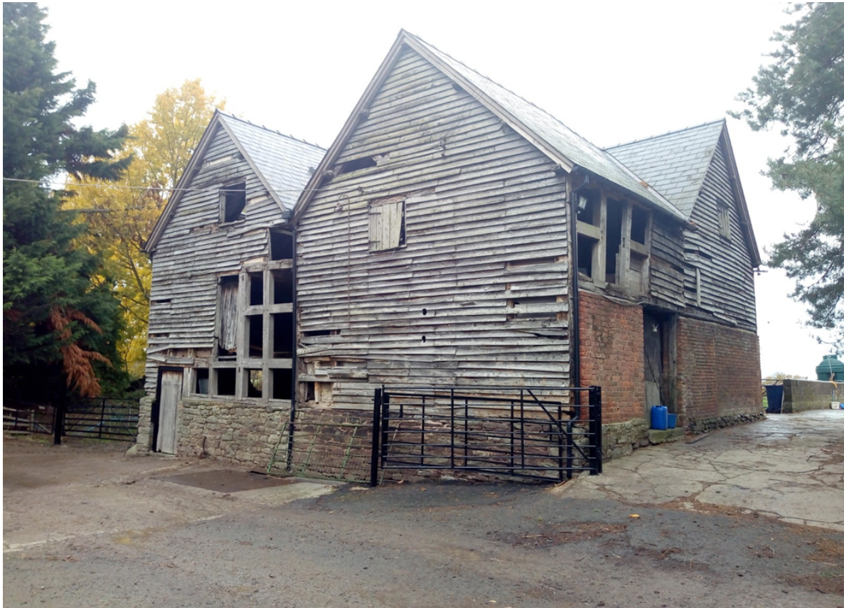
Figure 5: Existing barn to the north-west of the farmhouse
